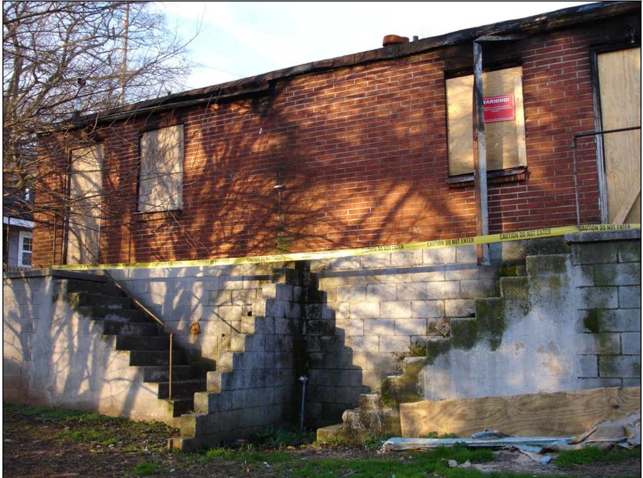
Photo 2. Rear (C-side) of incident structure. (NIOSH photo.)
